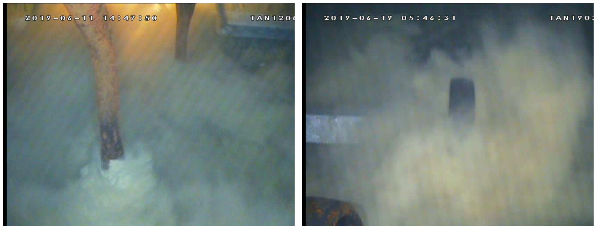
Figure 4-11: Images from the video cameras mounted on SCIP showing the tyne penetration (and roller) (left) and the sediment cloud being generated (right).
